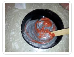
4. Combine Newtech Repairer and Red Hardener. Mix well to a uniform colour (no grey and red streaks visible).
